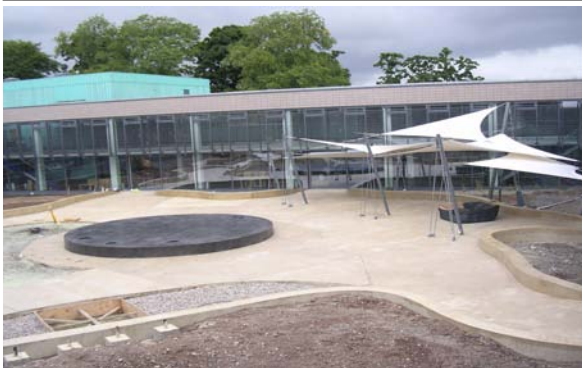
Above: The courtyard under construction
