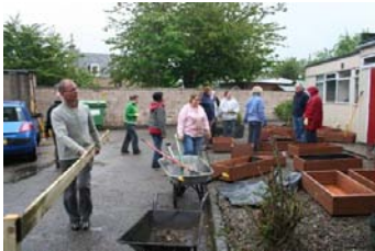
Above: A work in progress
