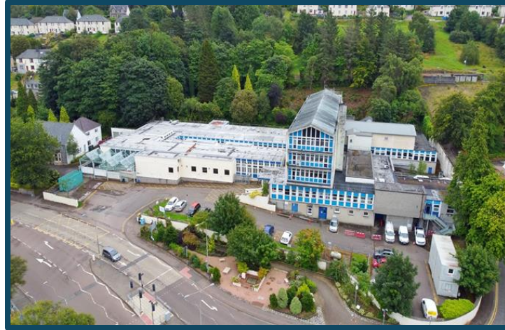
Above: External view of Belford Hospital
